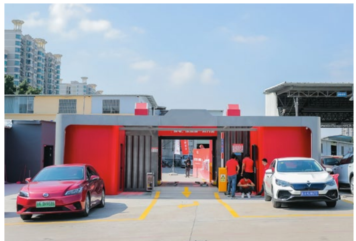
Aulton Dianba Batteriewechselstation 4.0
