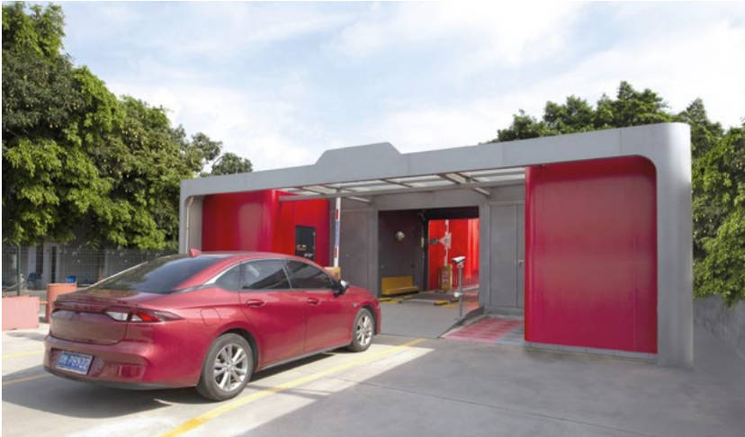
Aulton Dianba Batteriewechselstation 4.0
